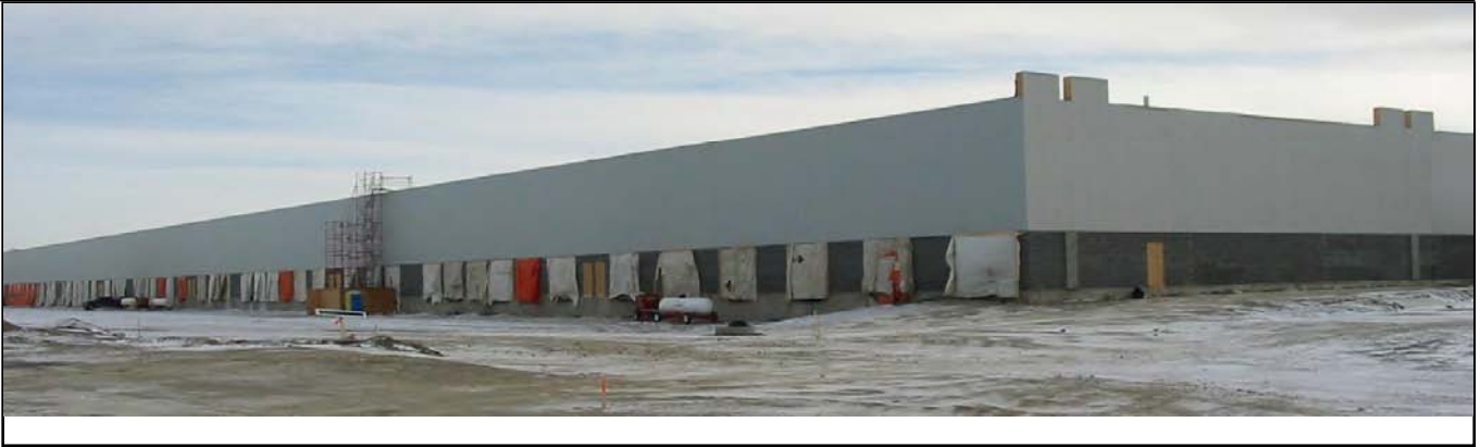
Warehouse Application 350,000 SQ FT_ 28 FT Ceiling 9.8 Million Cubic FT.
