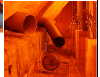
TRENCH 200' X 10'W X 6'D 3' of Frost in 4 days
